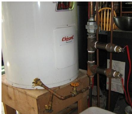
So why is this so good? With a thermostatically controlled output, the water leaving the heater is maintained at the temperature of the thermostat. This means that the varying heat
